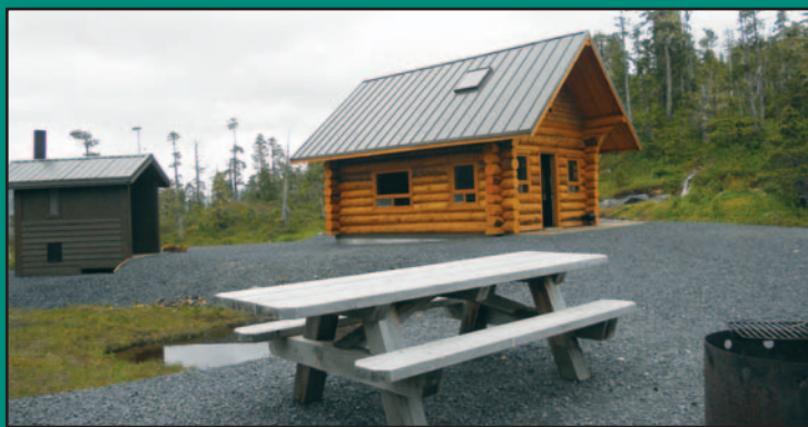
The Middle Ridge Cabin is the Wrangell Ranger District's first road accessible cabin. The cabin is about 20 miles outside of town and is accessible to high clearance vehicles in the summer and snow machine, snowshoe and ski in the winter.
